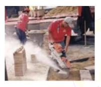
Use saw equipped with integrated water delivery system that continuously feeds water to the blade.
