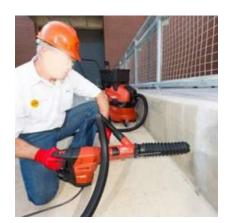
Use drill equipped with commercially available shroud or cowling with dust collection system
