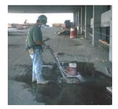
Use saw equipped with integrated water delivery system that continuously feeds water to the blade.
